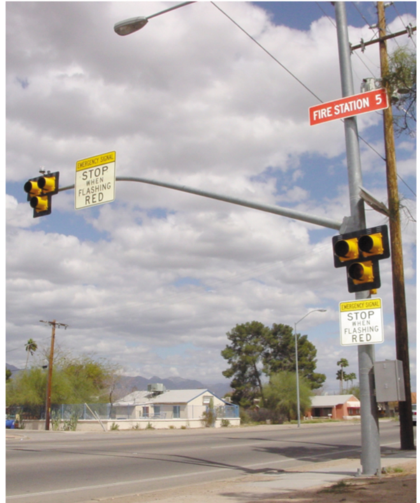
Tucson's Fire Station #5 with solar-powered flashing beacons.
