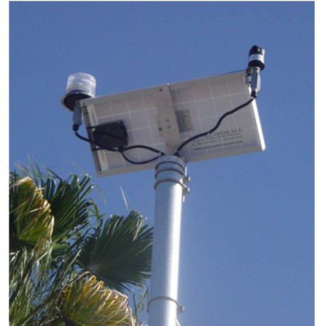
Close-up flashing beacon detector and confirmation light mounted to solar array.
