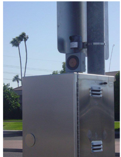
Close-up detector assembly
