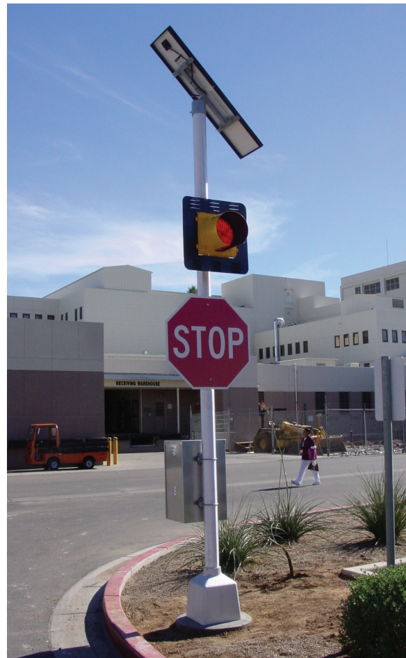
Figure 2: 40W solar flasher system at Phoenix, Arizona VA hospital.
