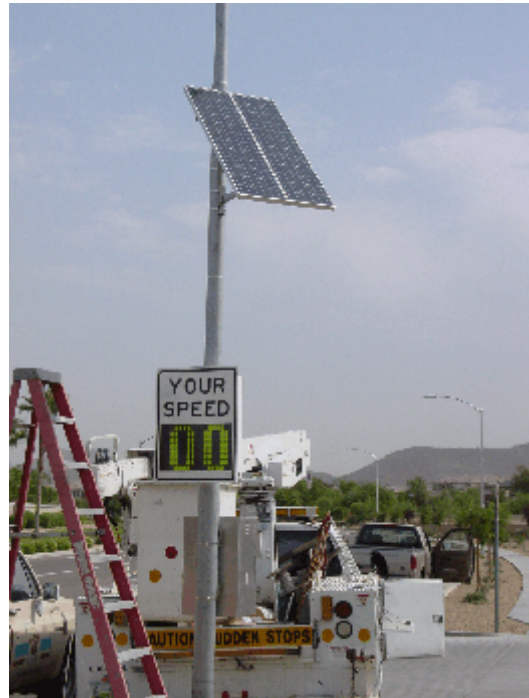
Installation of 3M DFB sign in Glendale, Arizona
