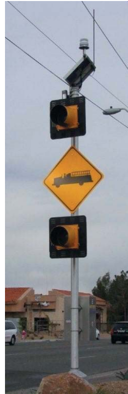
Figure 4, typical dual lamp flashing beacon systems. Right unit features the clear confirmation strobe.
