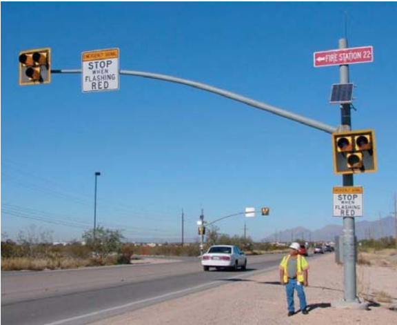
Figure 5, City of Tucson fire station exit signal with "Mickey Mouse" signal head.
