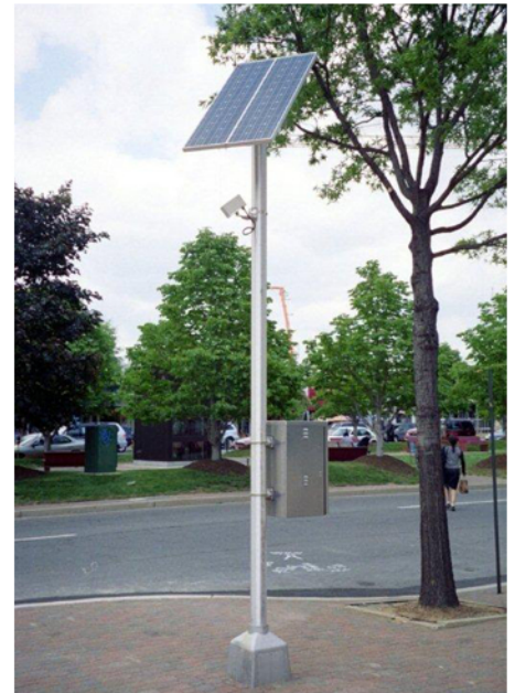
Sensor station for sensor-activated crosswalk flasher. Photo courtesy of Randy Dominick, Traffic Systems & Technology.
