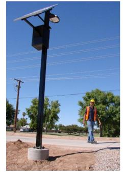
Due to the large number of systems fielded, STC designed field test equipment to minimize hookup errors. A handheld test module which plugs into the system wiring harness has been provided to field technicians. The test unit provides visual feedback on the polarity of the battery and solar array connections.
